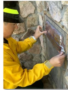
Applying vent tape
