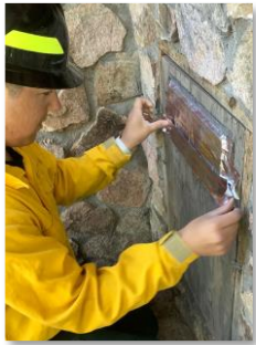
Applying vent tape
